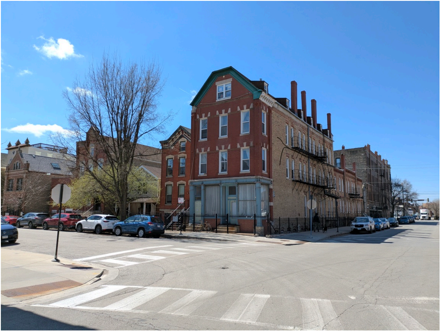
1362 N. Bosworth (Pulaski Park) (Corner building) Formerly 1362 Dickson Photo Credit: Michael E. Byczek. Copyright 2026.
