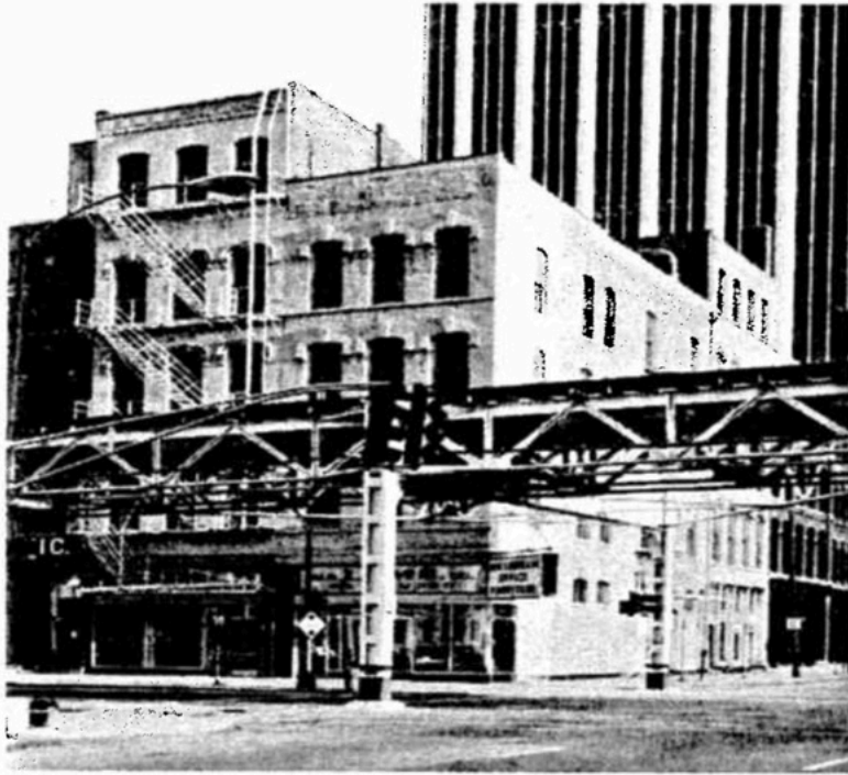
The Rowney Building is located at the corner of Lake and Franklin streets. One of its facades is partially obscured by the “L” structure—built 24 years after the building.
