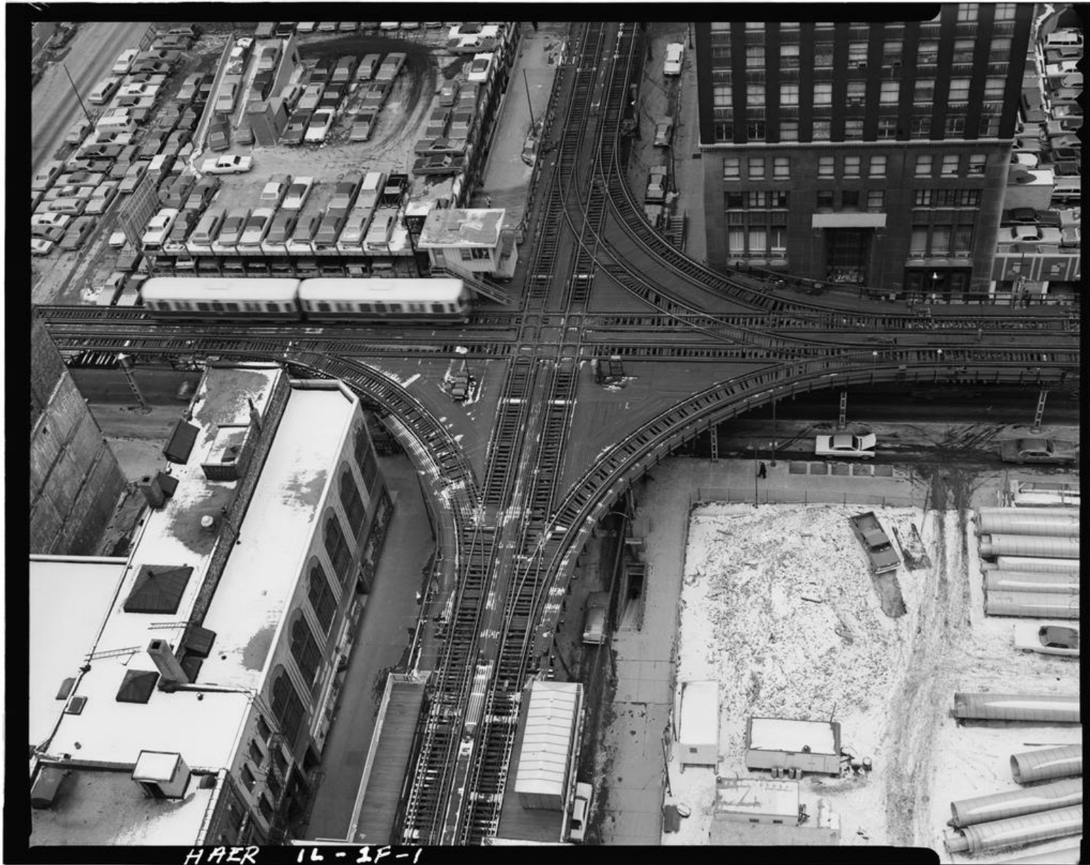
Another perspective that shows the William Rooney and Peter Ryan Building at the very bottom left corner of the photo [20B]
